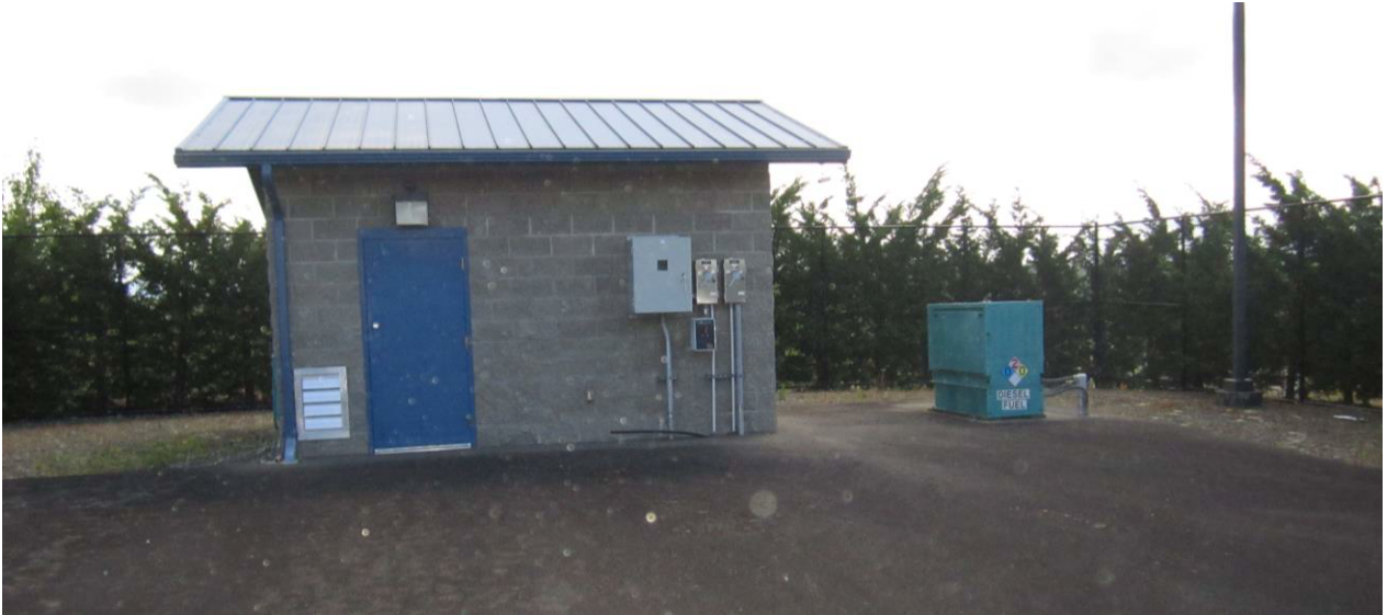
Panorama Heights Booster Pump Station
